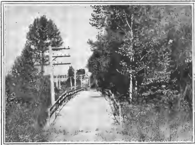
Old wooden bridge a few miles out of Winston-Salem on the way to Kernersville
